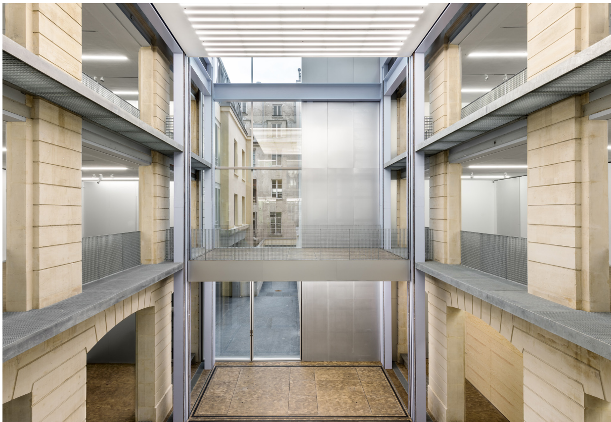
1.6 OMA, Fondation d'Entreprise Galeries Lafayette. Four movable platforms allow for multiple configurations of the building.
