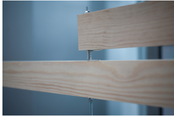
3.13 Mobile of planks, forming a wall. Detail of spring-loaded hinge.
