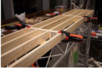
3.26 Mounting box frames to truss system.
