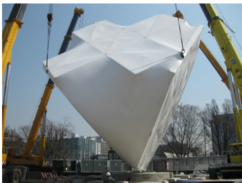
4.51 OMA, Prada Transformer. Four mobile cranes change its orientation.
