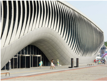
1.4 soma, One Ocean Pavilion. 98 flexible louvers in the external facade open and close to control daylight influx.
