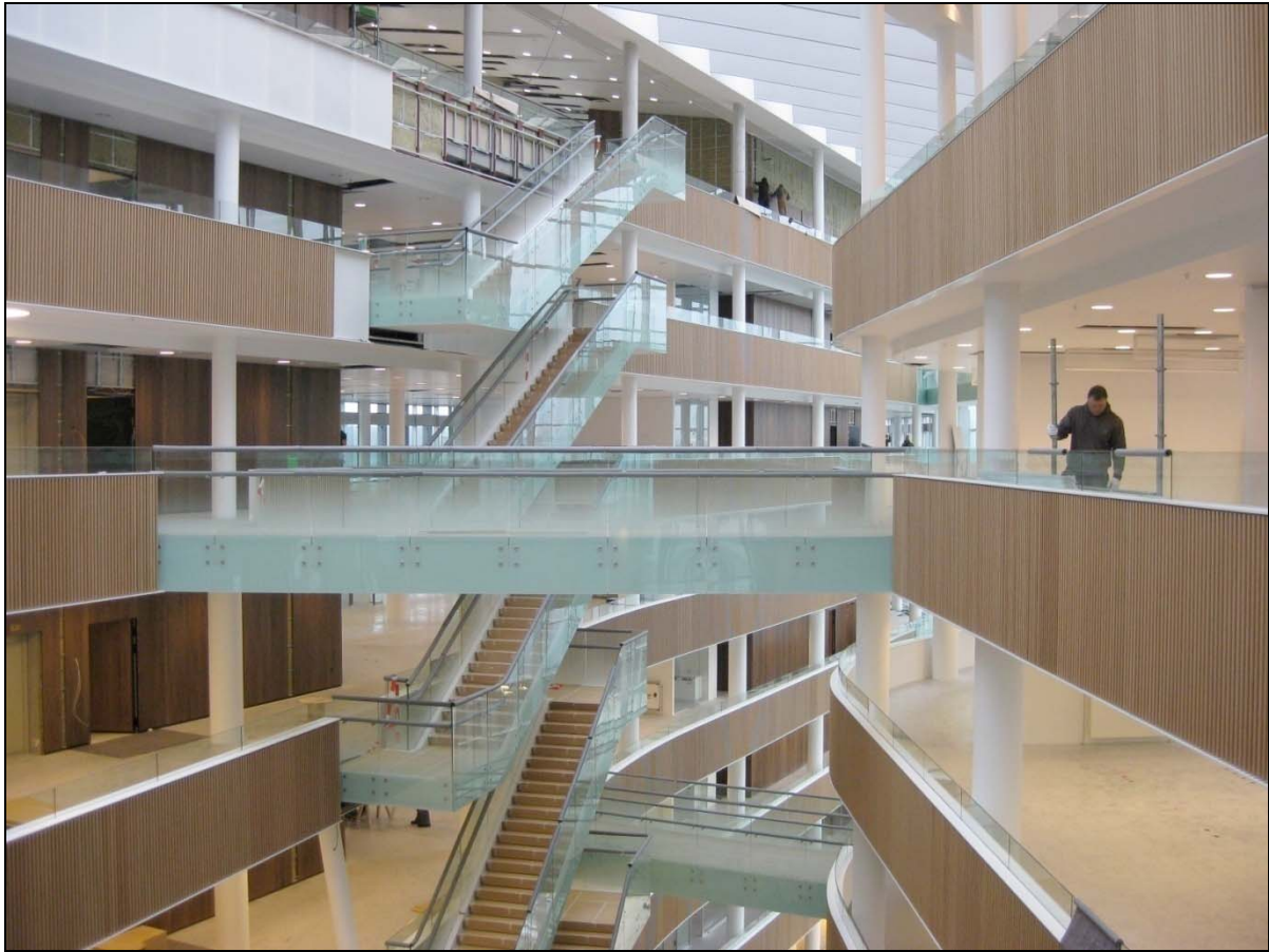
Figure 11: Inside the domicile building under construction.
