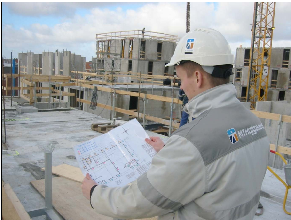
Figure 13: An engineer on site with an architectural plan in his hands.
