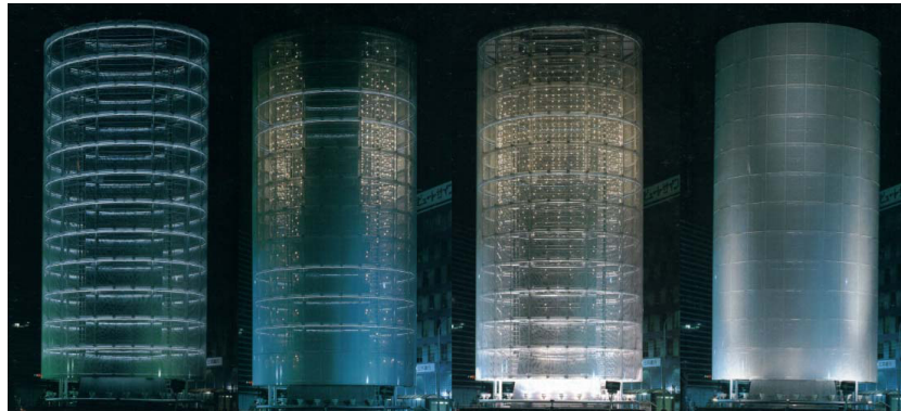
Figure 11 The Tower of Wind by Toyo Ito is a sculpture completed in Tokyo in 1986. The tower is a metaphorical representation of Tokyo with its ever-changing never-ceasing winds. The tower changes expression in response to winds' speed and directions (Photos with courtesy of Shinken-chiku-sha).
