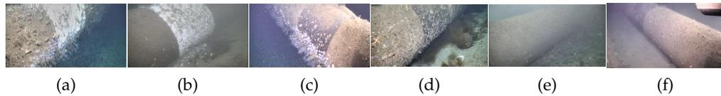
Figure 5.2: Example of the pipeline dataset: (a-b) an anode and pipeline, (c) a pipeline and a field joint, (d) a field joint, boulders and pipeline, (e) a pipeline alone, and (f) a pipeline, field joint, and part of a vehicle in the top right (best viewed in color).
